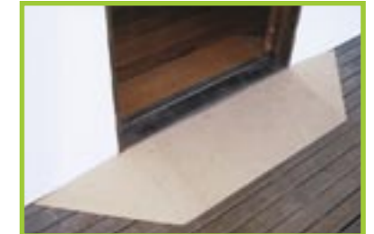
Timber wedge built by tradesperson
